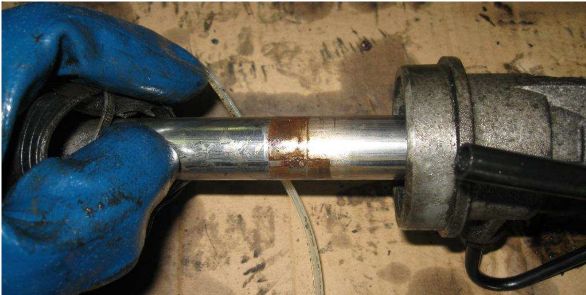
NOT GOOD - Rusty rack
